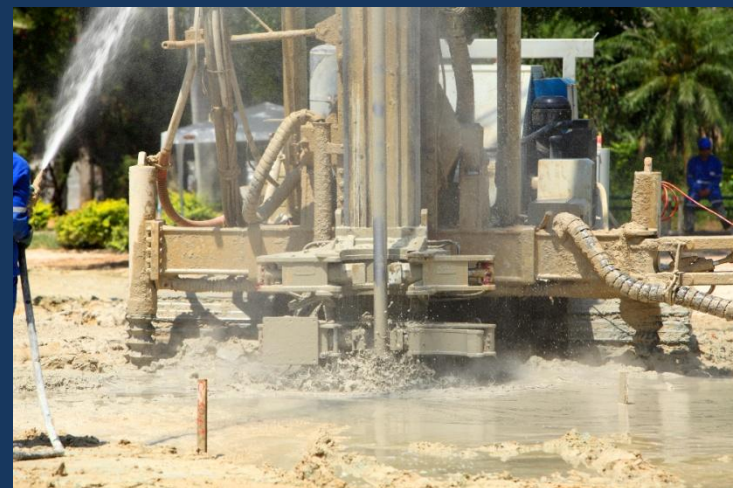
O Jet Grouting impermeabiliza o solo
