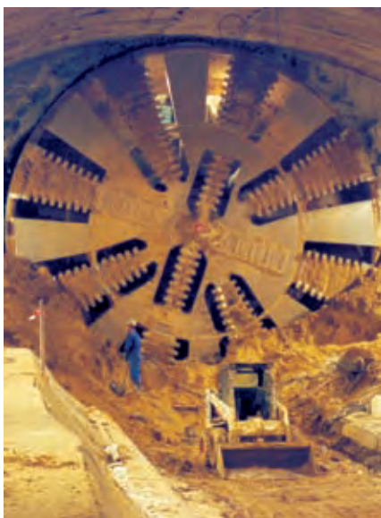
Tunnelling machine entering a Metro station
