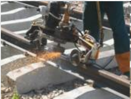
Rail grinding
