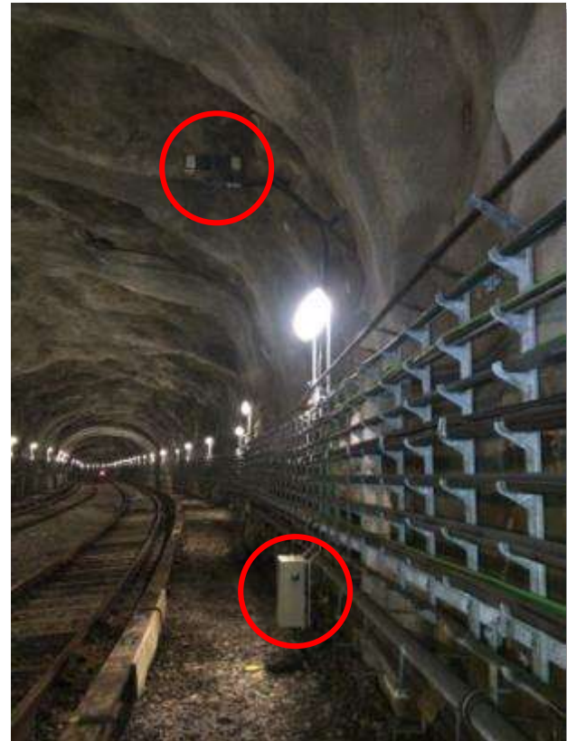
Track side Antennas and interface box
